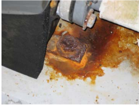
Anchorage Deterioration
