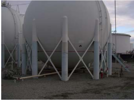
Remediated Bracing On Spheres
